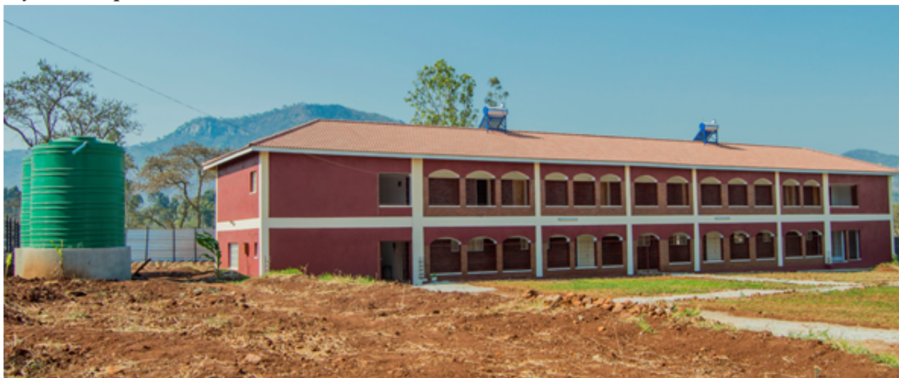
The newly constructed Monastery of Holy Name located in Weirmouth in Mutare.
